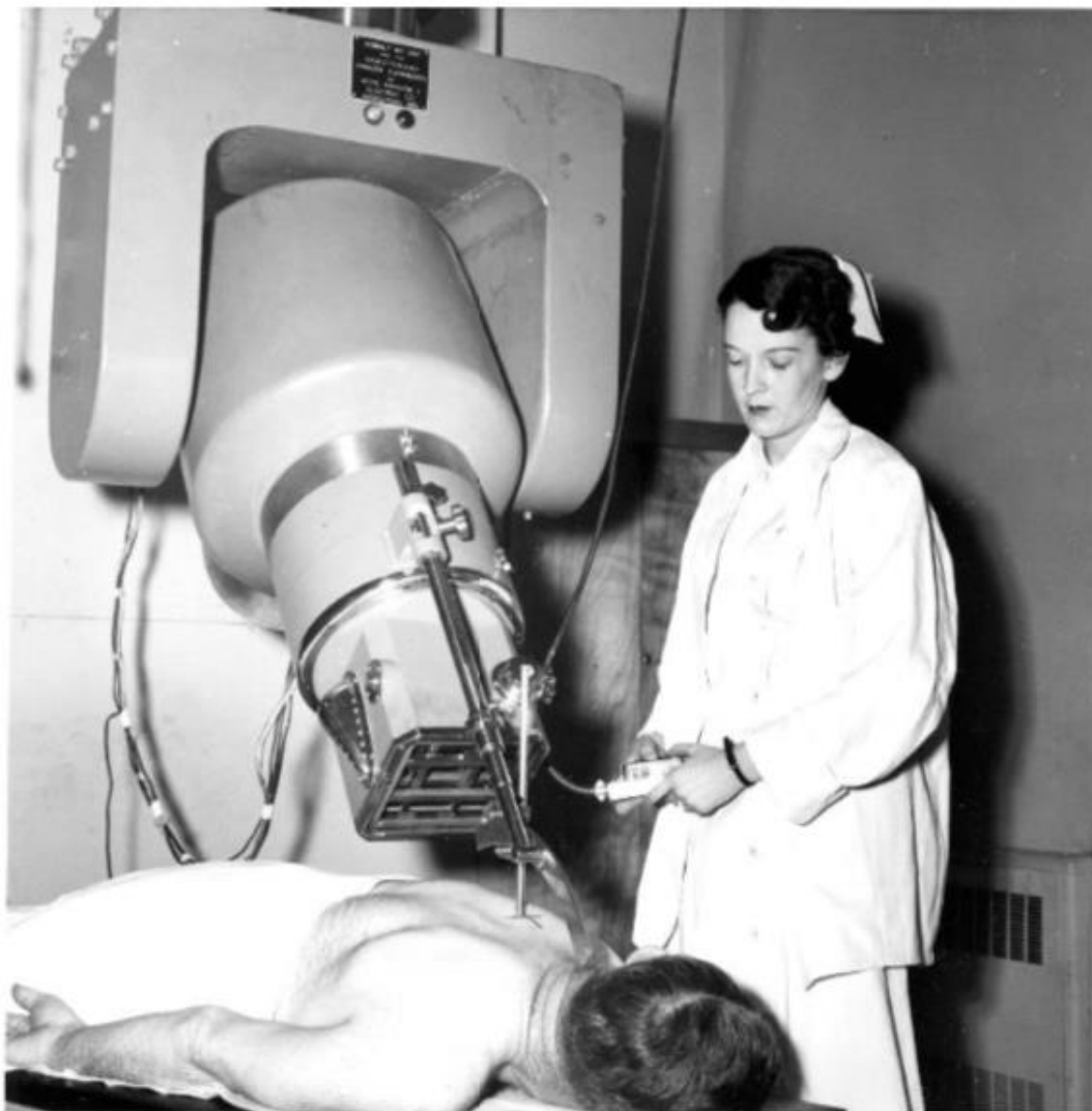
Figure 2. The Saskatoon Unit designed by Harold Johns and students, and John MacKay of Acme Machine and Electric of Saskatoon. From University of Saskatchewan, University Archives and Special Collections, University Photograph Collection, A-2244.
