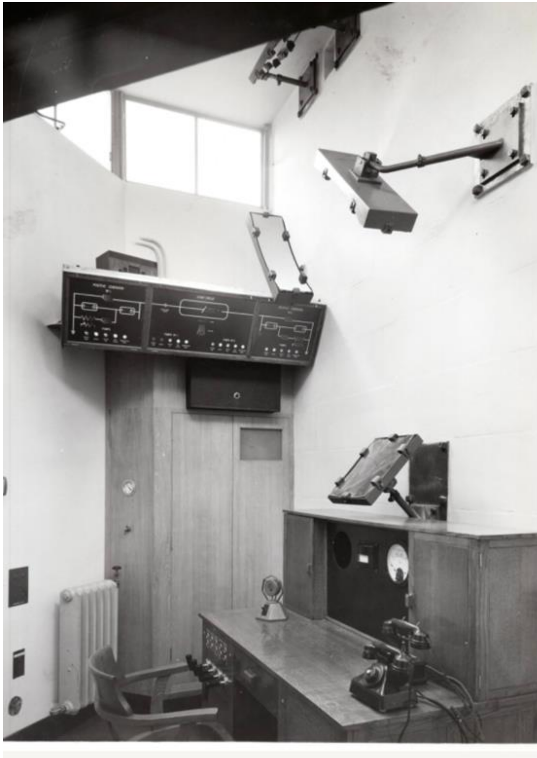
Control Room showing: Dose rate meter; microphone (communication with patient; simple circuit diagram with lights to show any faults; the periscope system of mirrors to view the patient on the other side of the barrier)
